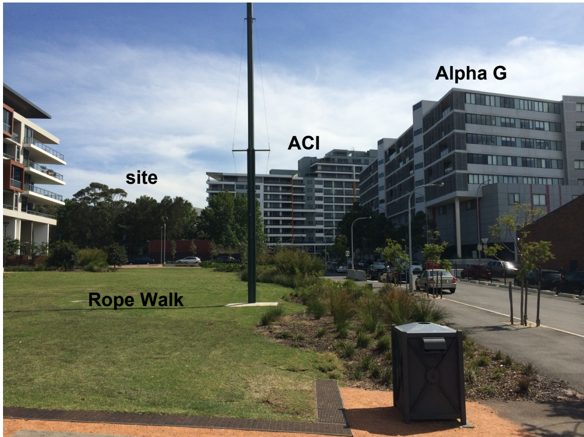
Figure 11: Rope Walk park, ACI and Alpha G, viewed from Archibald Avenue in a northerly direction.
